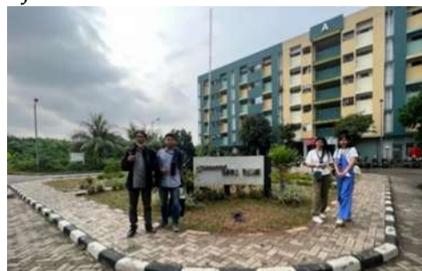
Figure 1. Rawa Bebek Rental Flats Building
