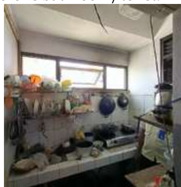
Figure 6. Window Opening in the Flats Unit
