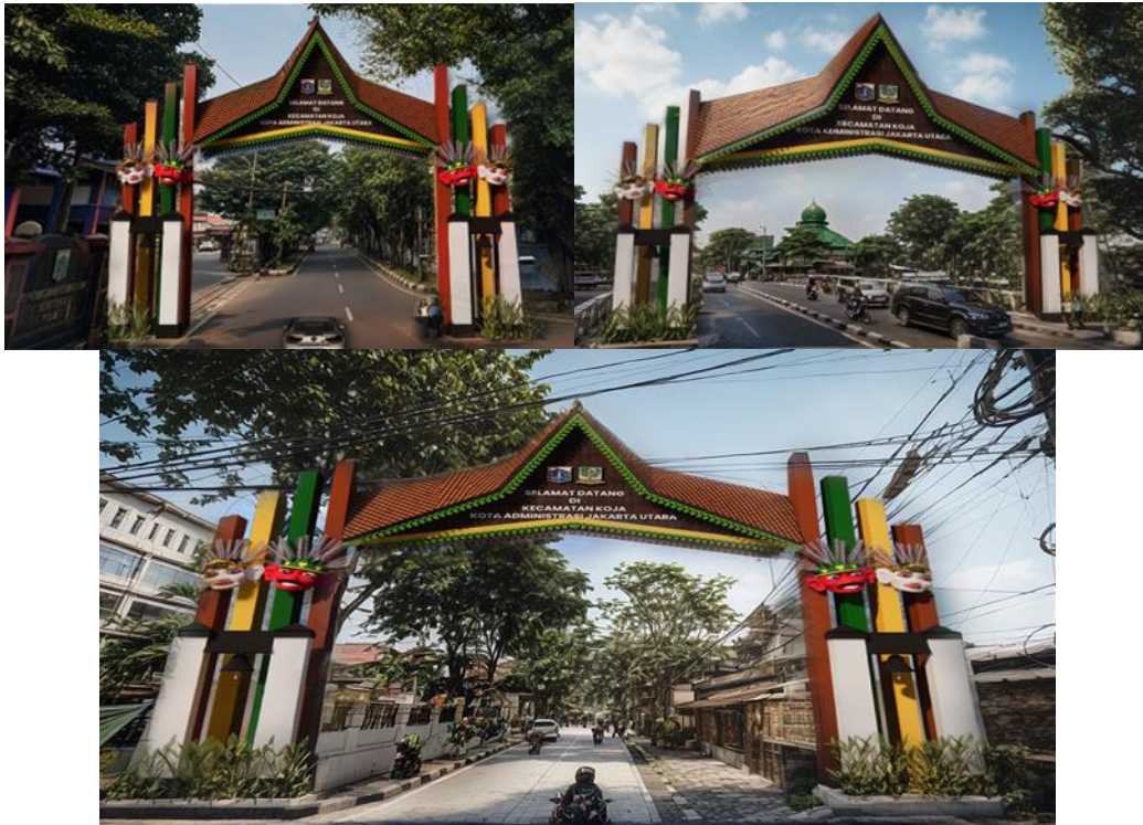
Figure 7. Results of the Gate Redesign at the Koja District Office, North Jakarta Administrative City
