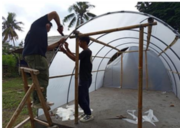
Figure 1. Construction of the Drying House
