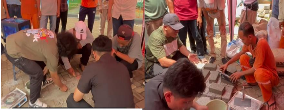
Figure 8. Paving Block Mixing and Molding Process using Plastic Material Mixture
