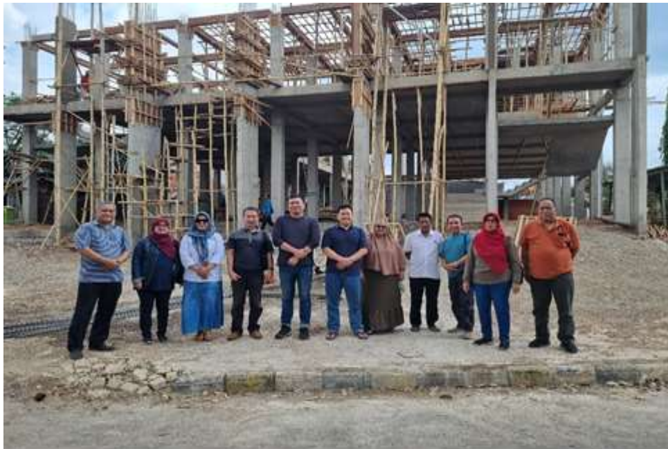
Figure 4. Actual Condition of the Mosque Under Construction
