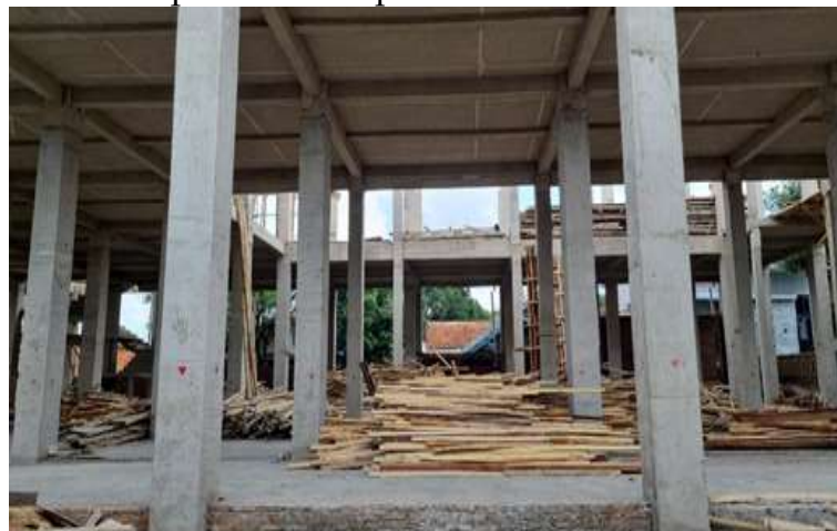
Figure 1. The Mosque Under Construction
